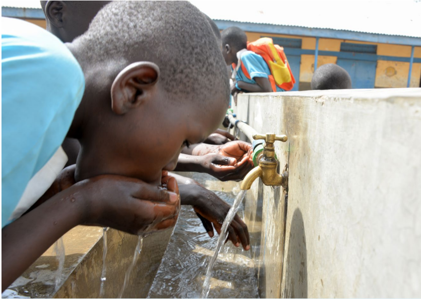
Pupils of Amelo Primary school in Adjumani District drink safe and clean water from taps in the school compound. The water is pumped from a solar powered water system constructed under the Water, Sanitation and Hygiene (WASH) project with funding from the Government of the Republic of Iceland © UNICEF Uganda
