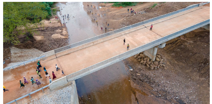
Nyara Bridge in Terego District, West Nile Sub-region ©UNOPS Uganda
