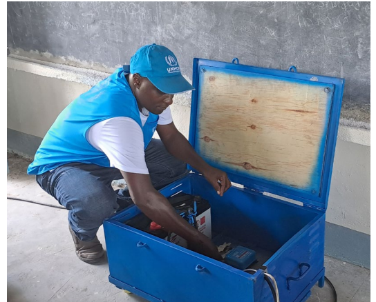
John Paul Ojok attending to the solar power box ©UNHCR Uganda
